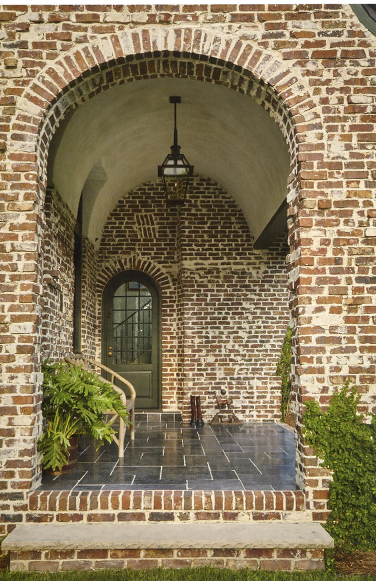
ABOVE Architect Peter Block used aged clinker bricks with custom mortar, giving a nod to the Low Country vernacular.
